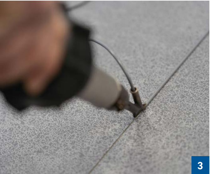
Hot cord welding
