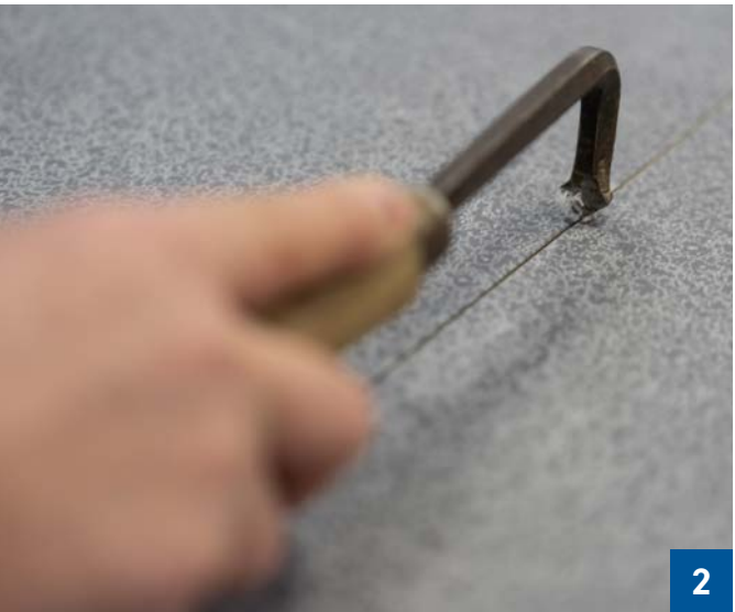
Grooving before welding
