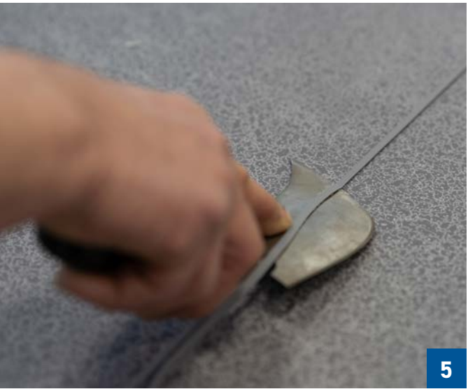
Second and final cord trimming
